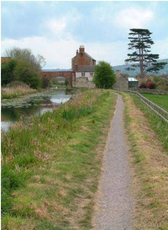
Conservation areas are designated to protect the character of an area in all its aspects. These are attractive houses in their own right but it is the relationship between them, the bridge, the boundary walls, canal, trees and the open landscape setting which together is so special.
